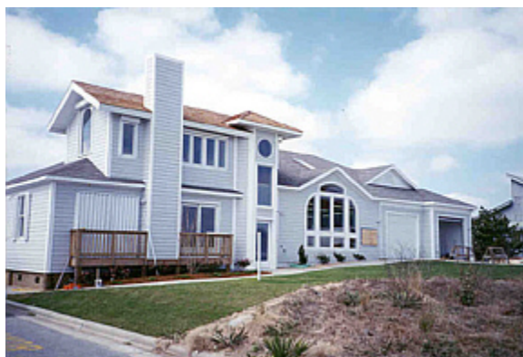
Figure 2.1. Two-story test house located in Southern Shores, N.C., used by Jones and Porterfield (1999)
